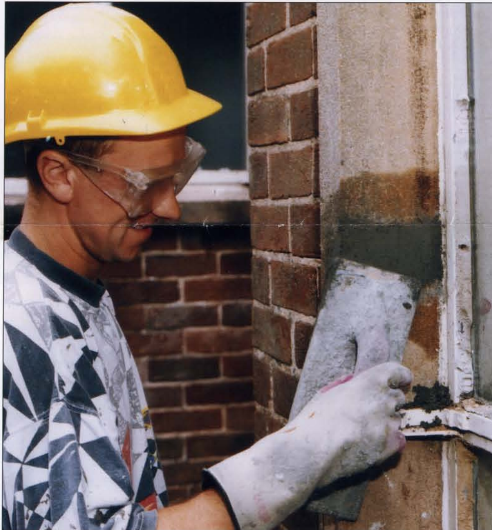
Concrete repair projects demand specialist capabilities
