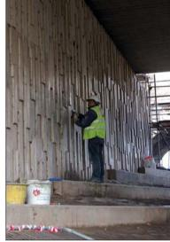
Extensive concrete repairs, as well as the design and installation of electro-chemical works (permanent monitoring and cathodic protection trials) have been carried out at Cliff Gardens Bridge, in Old Colwyn, by CRA member Quadriga Concepts Ltd.
