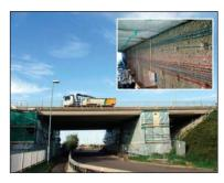
Principal Inspection reports on the two bridges at Tipner Interchange in Portsmouth revealed leaking joints above the two intermediate piers on each structure. Subsequent testing work confirmed the presence of very high chloride concentrations in the piers.
