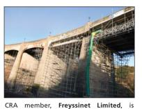
currently working on a £1.5m contract for repairs to the A92 Jubilee Bervie Bridge near Montrose, Scotland. This 1930s reinforced concrete structure has suffered the ravages of the marine environment and extensive repairs were required.
