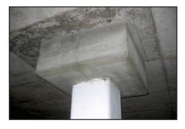
Work to column heads may involve using pre-bagged fluid flow materials to increase column head dimensions. This requires a very exact regime to ensure that the load from the slab is correctly 'picked up', through the precise location of new reinforcement and attention to detail in the production of the necessary formwork.
