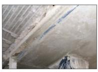
CRA manufacturer member **Saint-Gobain Weber** supplied innovative spray concrete repair products for the permanent remedial repair of the Deansbrook Viaduct.
