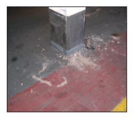
Corrosion of reinforcing steel results in the loss of steel cross-section, which may significantly restrict load-bearing capability and may lead to punching shear issues in the area of the columns.
