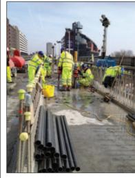
The Hammersmith Flyover, an elevated roadway in west London which carries the A4 dual carriageway, was closed just before Christmas 2011 after inspections revealed a significant corrosion problem with the existing post-tensioning installed in the early 1960s.
